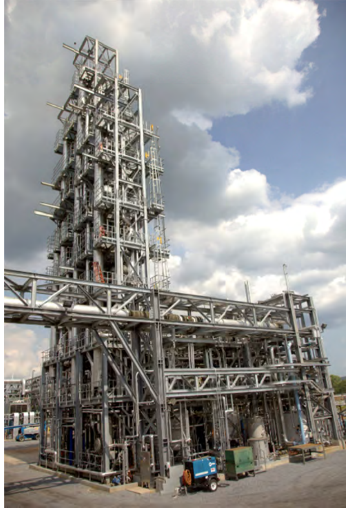
FIGURE 3.6 Conventional amine solvent plant for CO 2 separation at the National Carbon Capture Center in Wilsonville, Alabama. This is a demonstration plant that bridges technologies from the bench-scale to pilot scale, and the absorber unit that is currently in place captures 3,650 tCO 2 per year. In contrast to the air contactor used for extremely dilute air capture, this flue gas contactor (absorption column) can be tall for increased CO 2 separation due to the inherent driving force of the flue gas stream. This image provides an example for dimensional comparison to the DAC plant in Figure 3.5, not a comparison of scale as the annual removal rate by the National Carbon Capture Center is small since it is for demonstration purposes only. SOURCE: Courtesy of Frank Morton, Business Development Manager of the National Carbon Capture Center, Southern Company.
