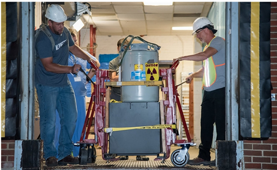
FIGURE 7-1 Workers remove a cesium-137 irradiator from Medstar Georgetown University Hospital in 2018. Efforts such as this have been highly effective in decreasing the number of at risk radiological sources in applications where safer alternatives are available.
